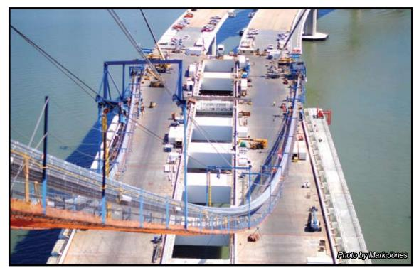
Shown from the top of the 525-foot single tower, the main cable for the new Bay Bridge East Span measures 2.6 feet in diameter and is comprised of 137 hexagonal strands
